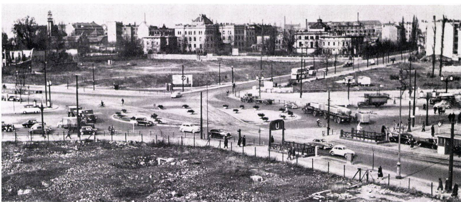
6 Tangenten um die City. Tangents autour du noyau de la capitale. Tangents around the City.
