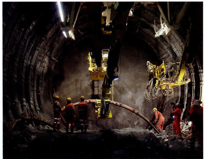
... to make the first breakthrough on 6 September 2006.
