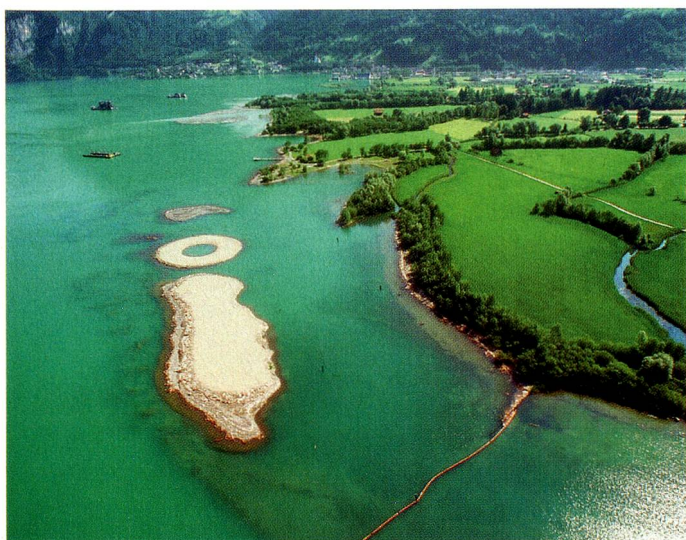
Filling with excavated material from the Gotthard in the Reuss delta near Flüelen.
