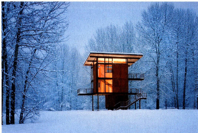
The Delta Shelter, a weekend cabin located on the flood banks of the Mazama River in eastern Washington. Because of seasonal flooding, the entire cabin was raised off the ground on stilts, which also heightened the 360-degree view of the natural setting.
