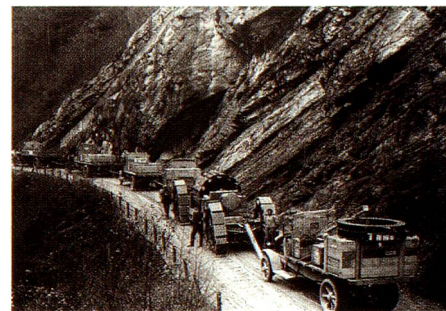
Industrial history: Brown Boveri lorries transporting generator parts to Wägitalersee lake (1924)
