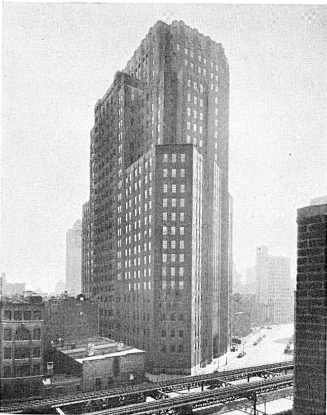
Fig. 13. «Long Lines Building» 32th avenue of the Americas, New-York
