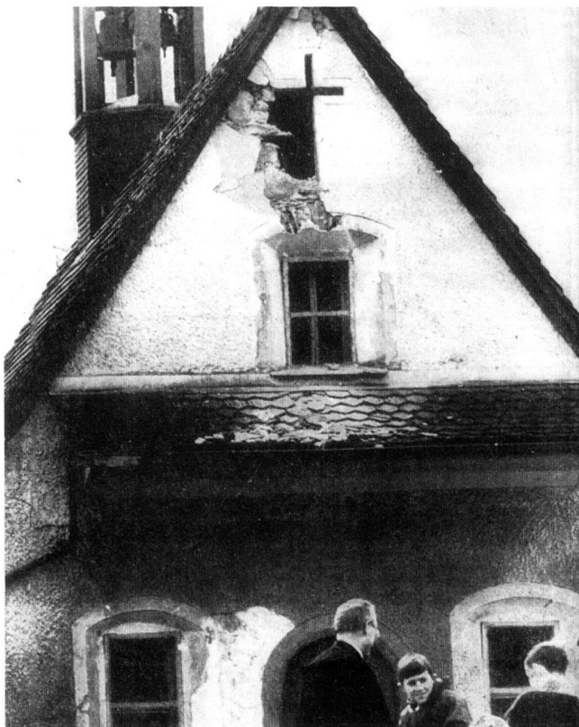
Fig. 10. Sarnen: A church, built in 1646, suffered heavy damage (Luzerner Tagblatt, March 16, 1964)
