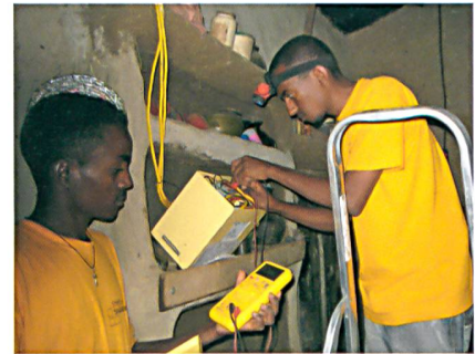
Installation eines Off-Grid-Solarsystems
