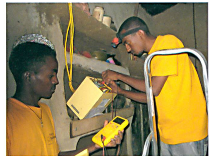
Installation eines Off-Grid-Solarsystems
