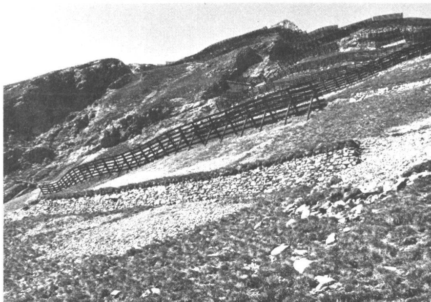
Fig. 6. The local sector DOL 6, intermediate sector on dolomite; anti avalanche defense works.
