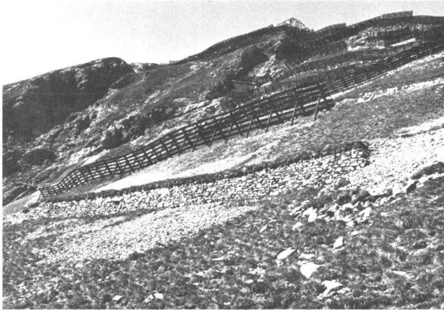
Fig. 6. The local sector DOL 6, intermediate sector on dolomite; anti avalanche defense works.
