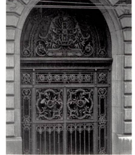
Bollwerkpost, Detail Tor
