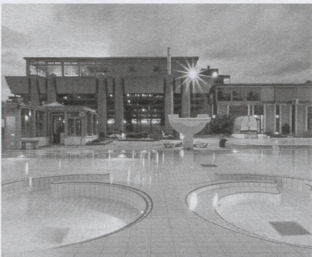
Thermal Centre at Yverdon-les-Bains
