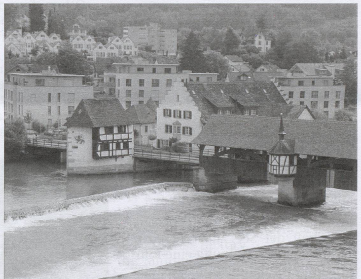
Old bridge in Bremgarten
