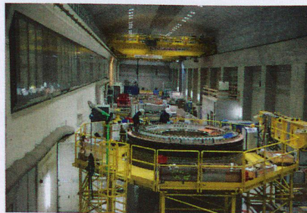
The so-called pumped-storage power plant generates or stores electricity by moving water between two mountain lakes separated by a 630-meter cliff.
