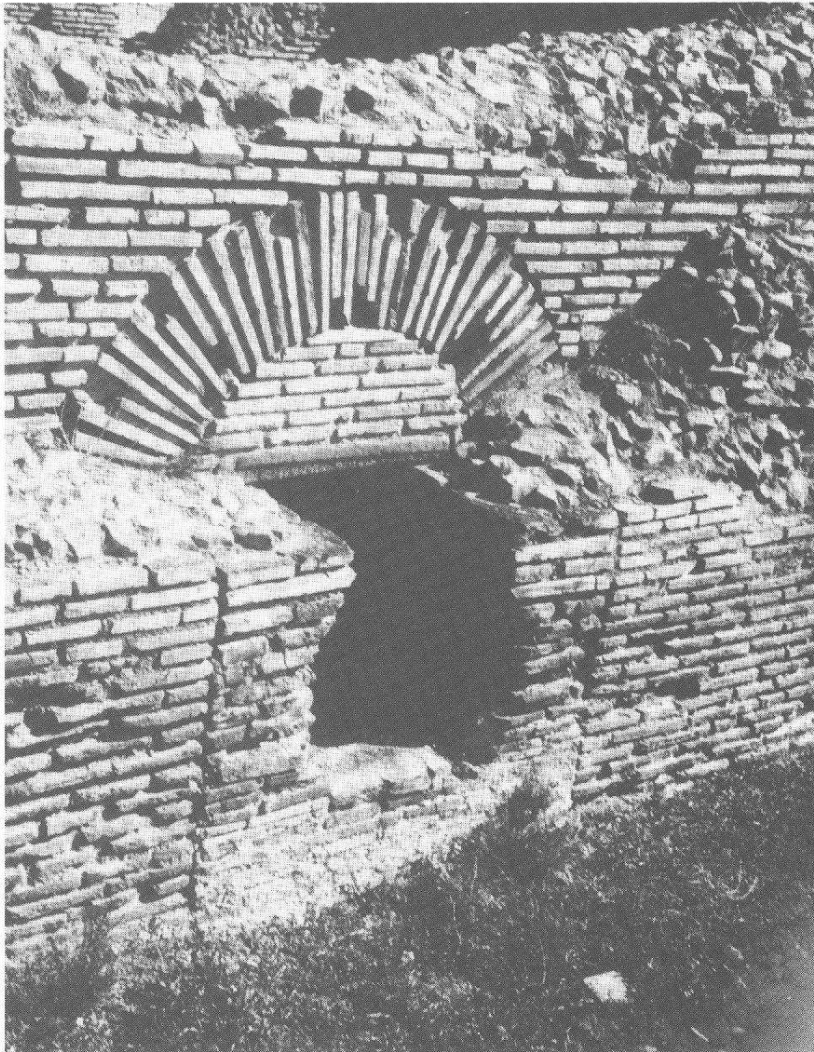
Abb. 2 Timgad, Praefurnium in den grossen Nordthermen.
