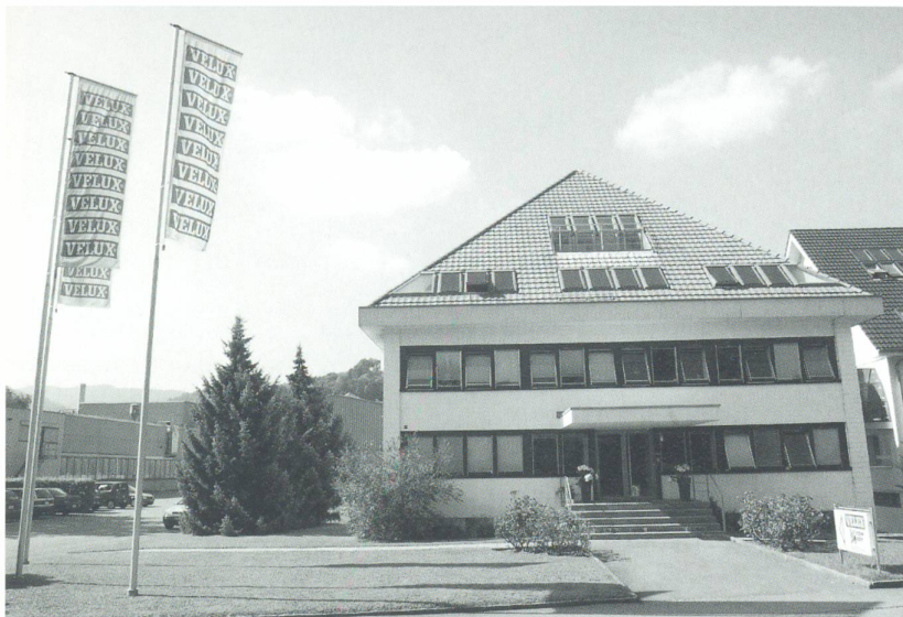
Velux in Trimbach
