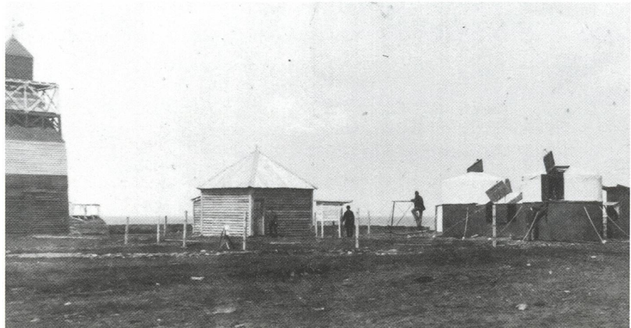
Fig. 7. Photograph of the German station in Punta Arenas. Left, wooden lighthouse of Punta Arenas, center, «tea house» and meteorological station, right, two observing domes made from iron and canvas (Archiv, Berlin-Brandenburgische Akademie der Wissenschaften).
