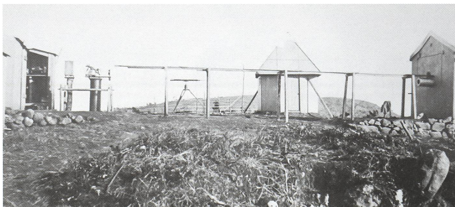
Fig. 3. The setup of the U.S. Nagasaki station in 1874 with a photoheliograph (no photographs of the 1882 observing stations are available at U.S.N.O.): On the left side, a pillar carries the heliostat; the solar rays are deflected by a mirror and pass through a lens and a small tube into a hut (at right) where the photographic plates are exposed (U.S. Naval Observatory photograph; courtesy of CHUCK BUETER).
