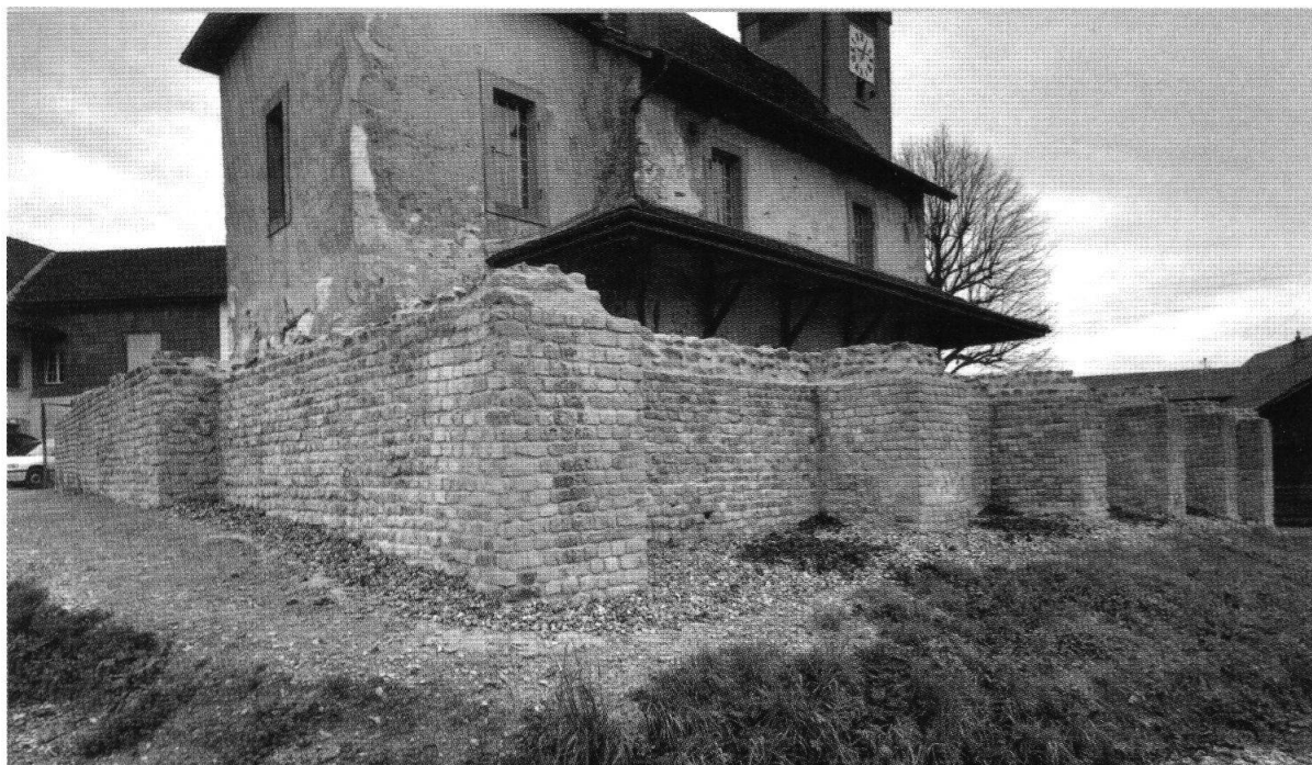
FIGURE 16 Ursins – Restauration des murs du temple gallo-romain. (Photo Fibbi-Aeppli)
