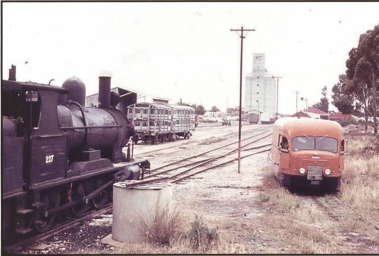
Taken in the late 1960s, a SAR Rx steam locomotive #227 with a Commer QX (R7) railcar #131 in the Karoonda rail yards. The petrol engine Commer railcar operated the Karoonda to Peebinga service. The grain silos in the background were built in the early 1960s employing an eight day continuous concrete pour.
