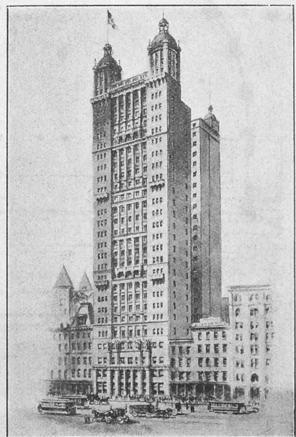
Abb. 17. New-York. — Park Row Office Building.
