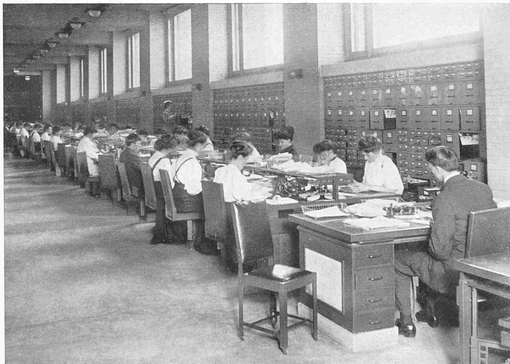
LARKIN BUILDING IN BUFFALO N. Y.
