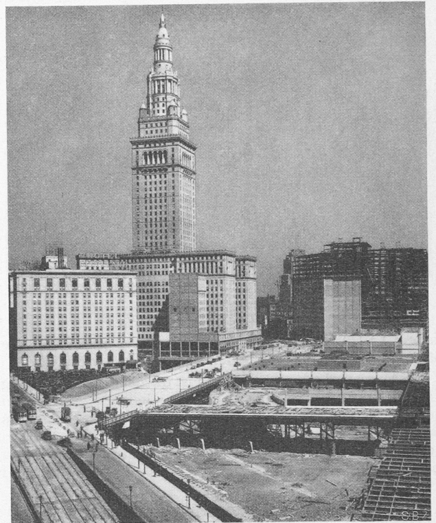
Abb. 22. Terminal Station in Cleveland.
