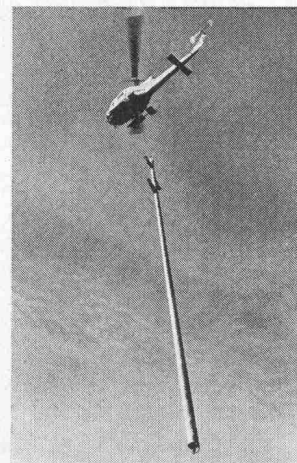
Transport eines 26-m-Mastes
