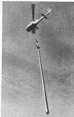
Transport eines 26-m-Mastes
