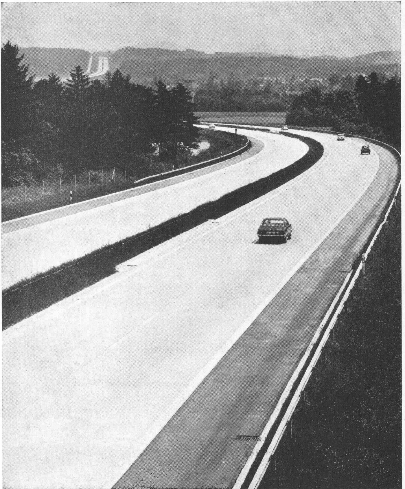
Nationalstrasse N 1 Wil—St. Gallen, Betonbelag
