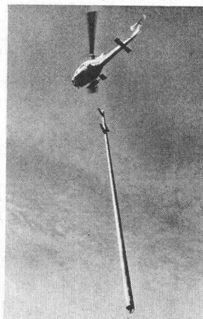
Transport eines 26-m-Mastes
