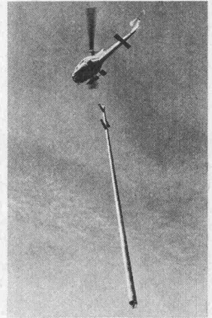
Transport eines 26-m-Mastes
