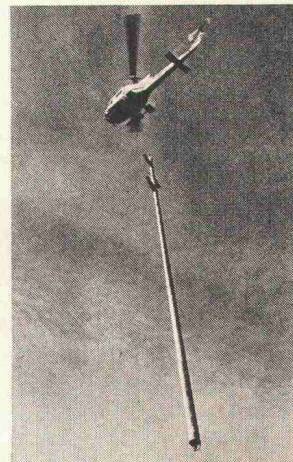
Transport eines 26-m-Mastes
