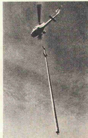
Transport eines 26-m-Mastes
