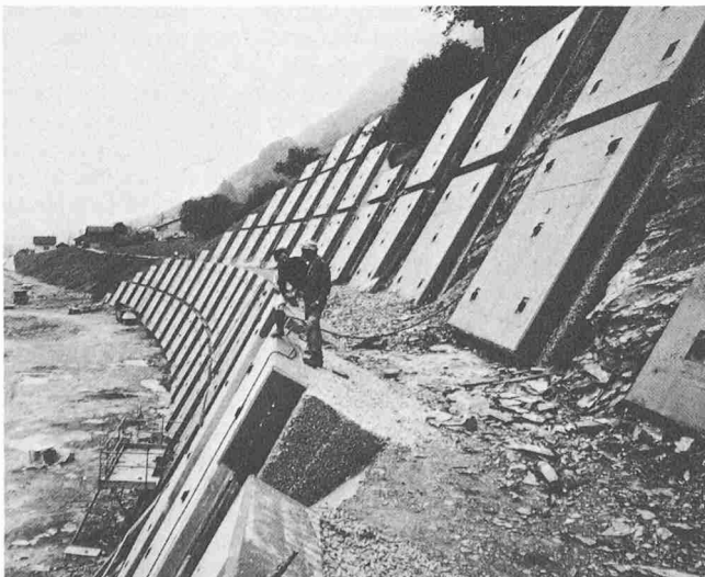
Fig. 18. Détail du Lot Bachmattli Detail of the Bachmattli lot
