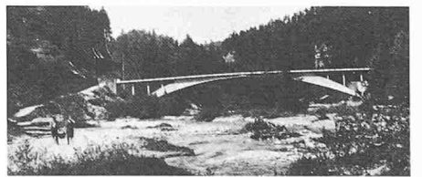
2051 Schwarzenburg 1932 Rossgrabenbrücke, Ing. Maillart Robert
