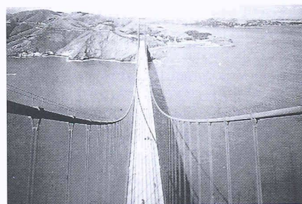
Golden Gate Bridge
