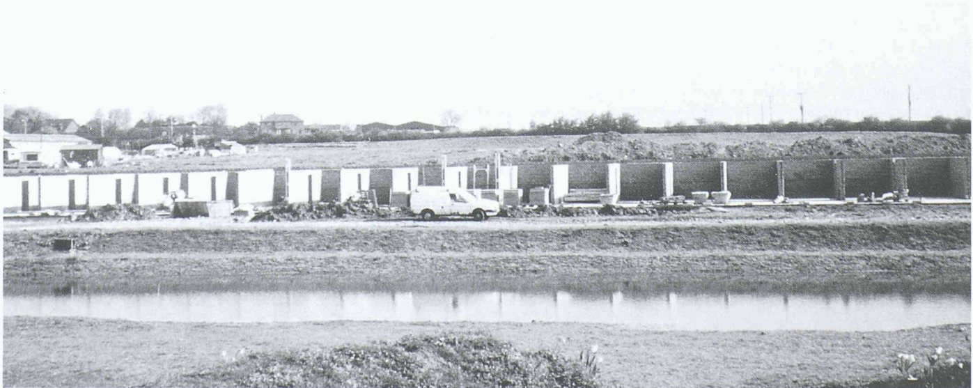
Hockerton Housing Project in der Grafschaft Nottinghamshire
