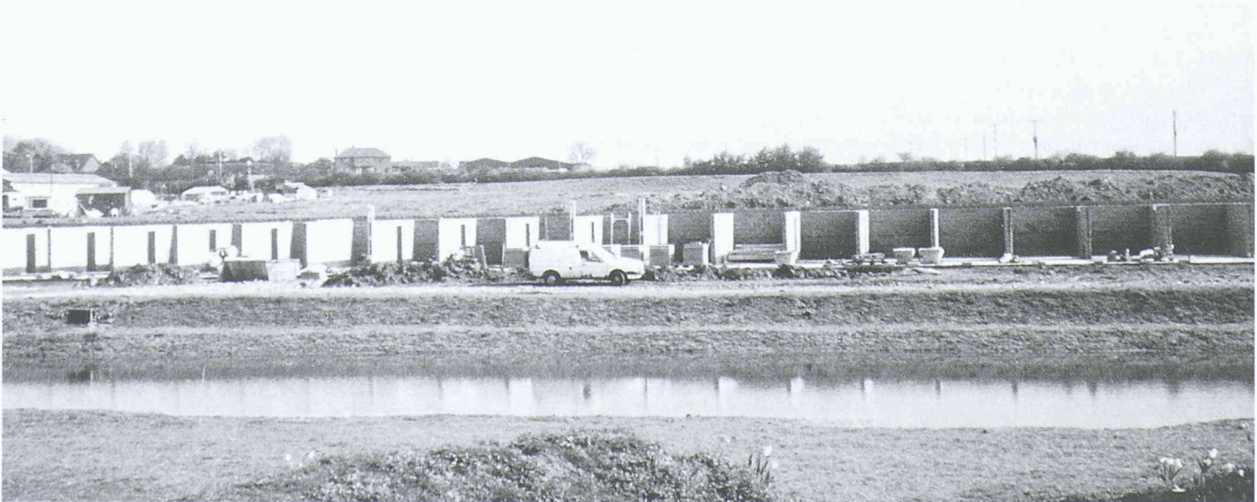
Hockerton Housing Project in der Grafschaft Nottinghamshire
