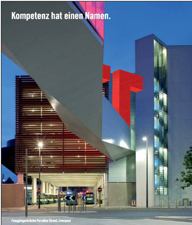
Fussgängerbrücke Paradise Street, Liverpool
