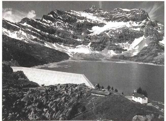
Staumauer Salanfe (VS)
