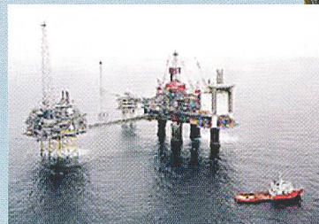
Sleipner platform (Courtesy STATOIL).
