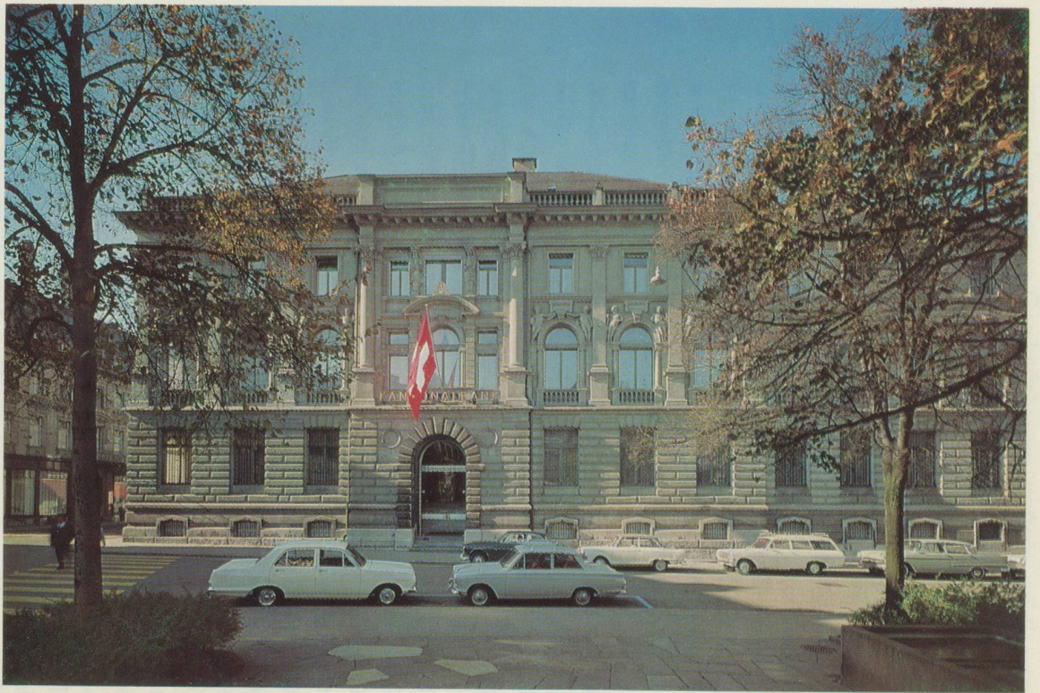
Hauptbank in St.Gallen
