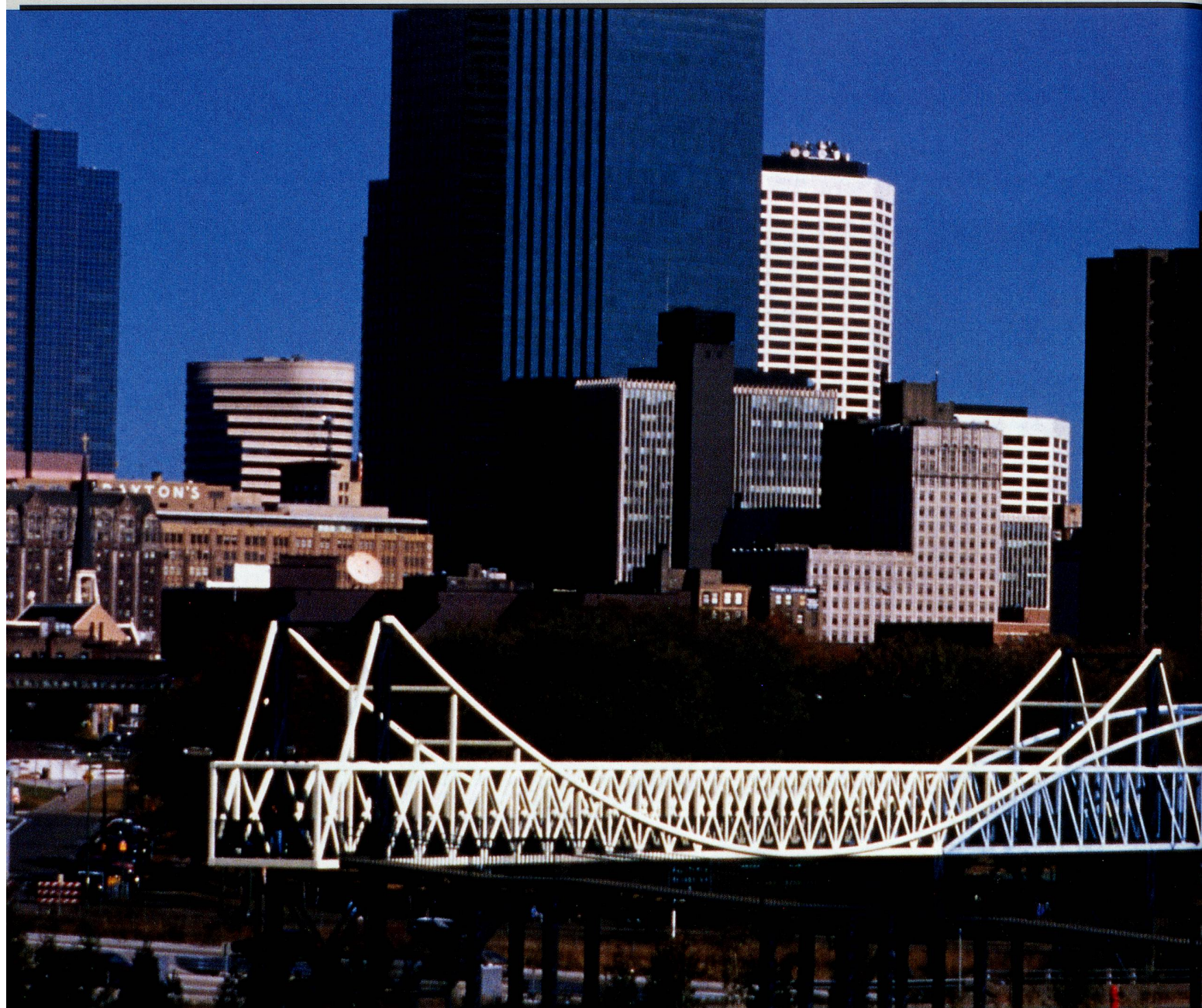
The Irene Hixon Whitney Pedestrian Bridge, 1988. Photo: MMK
