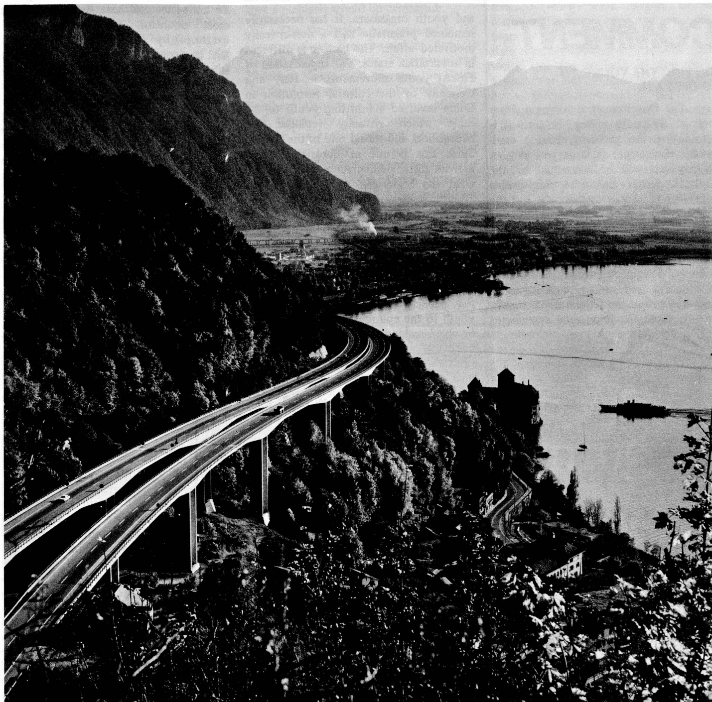
Bois de Chillon viaduct (1.4 miles) of the Swiss Motorway system above Lake Geneva. View of Chillon Castle and the lower reaches of the Rhone Valley with Lake Geneva.
