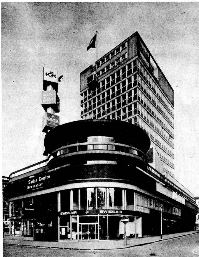
The Swiss centre towers high above the West End.
