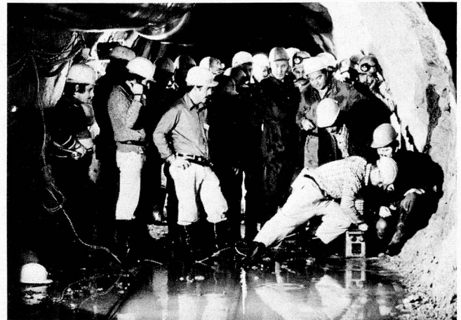
The Gotthard Tunnel is beginning to take shape – the last blasting.
