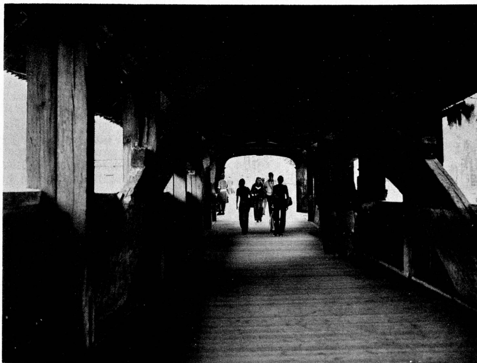
The Spreuer bridge is the less famous of the two wooden bridges across the Reuss. Up to the 16th century people were allowed to throw refuse into the river from here.
