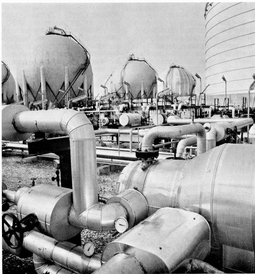
Storage facility with spherical tanks for petroleum gases, with refrigerant evaporators in the foreground.
