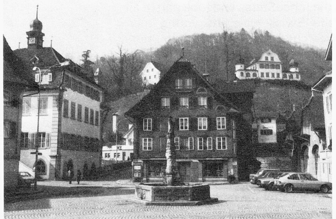
A square in the old Sarnen; on the left the town hall; the old shooting stand on the Landenberg hill (Photo Rheinhard).
