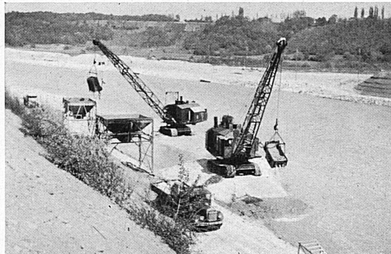
Draglines, 90 tonnes, 1 m³.
