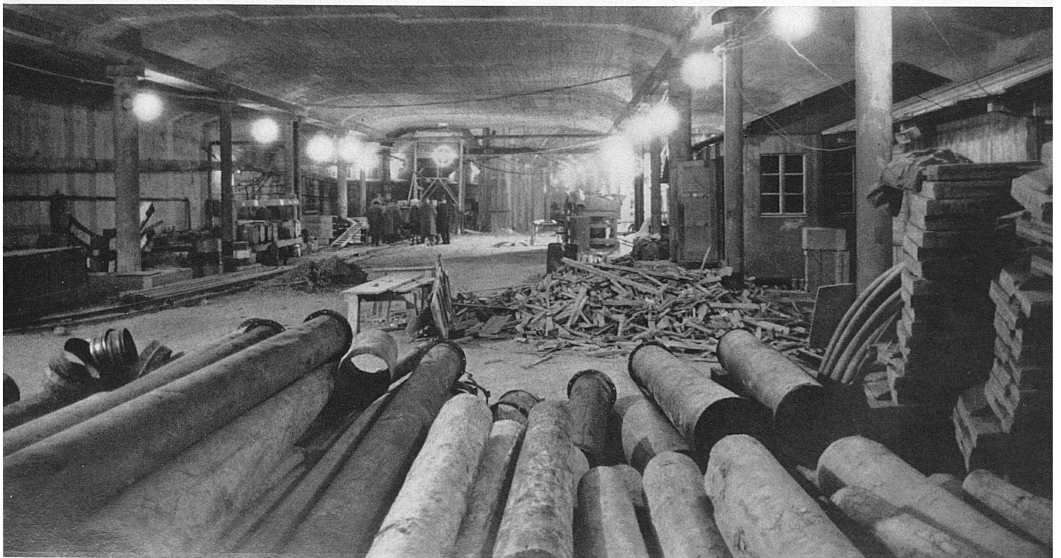
View of one of the special tunnels housing the cables required for the operation of a large electrified railway station.
