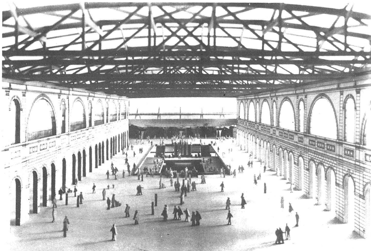
Improvement of stations. Zurich Hauptbahnhof main hall 1990. Photo SBB.
