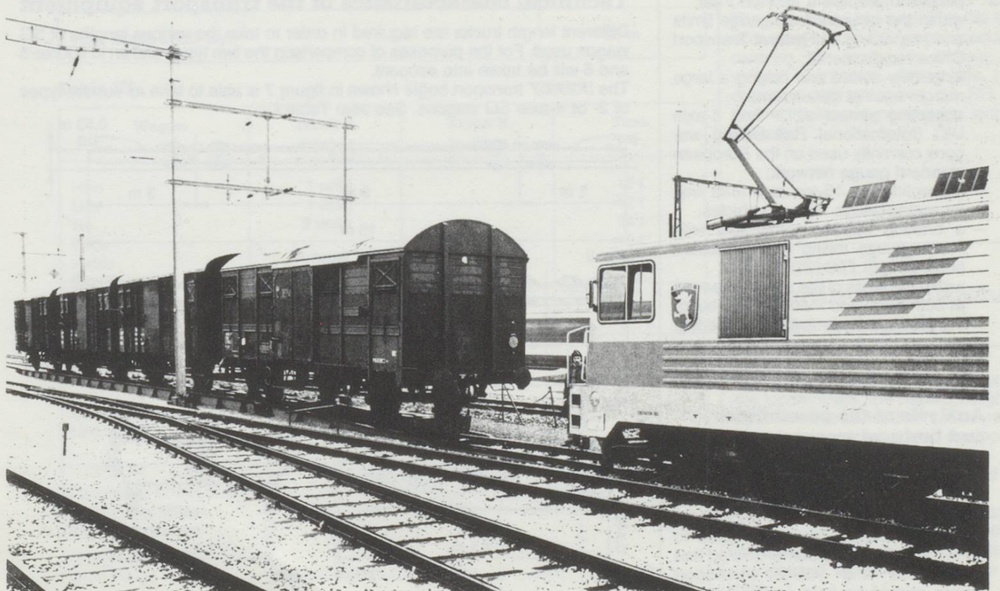
Fig. 2. The transfer station at Palézieux.
