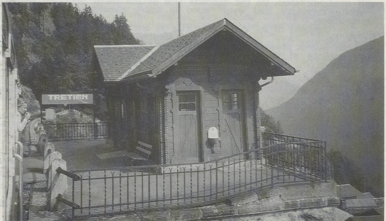
Below : Perched perilously on the mountainside, Tretien station on the Martigny Chatelard Photo Alan Pike
