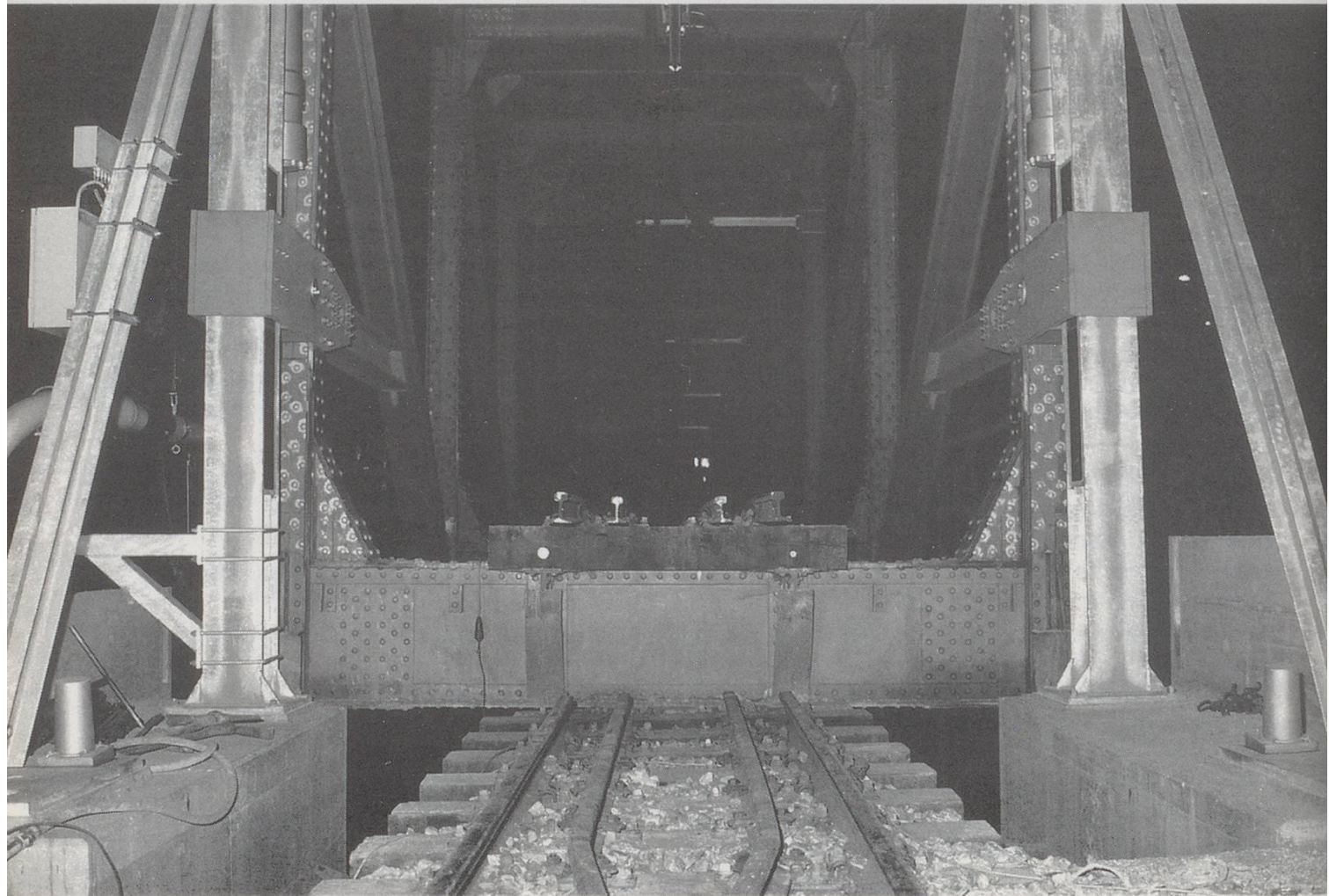
Furka-Oberalp Above & Below: Views of the bridge between Brig and Naters which now lifts so that if the river floods no damage will be sustained and rail connections can be maintained.
