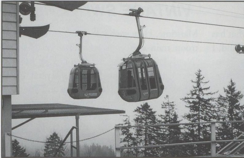
The top station at Fräkmüntegg on the first section of the cableway to Pilatus Kulm. May 2001. Photo: Editor
