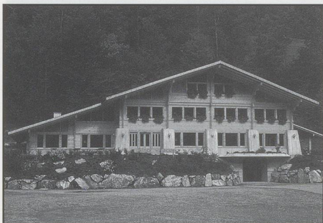
The Brienzwiler entrance restaurant at the Ballenberg Museum. Photo: Lester Weeks
